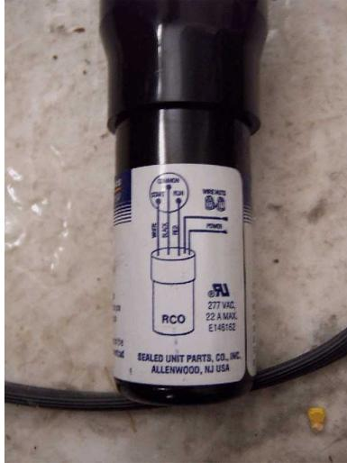
The terminal position shown on the 3n1 start relay diagram should match the compressor terminals. If the compressor terminals do not match the same position as the ones on the 3n1 start relay diagram just turn the diagram upside down so you have the single terminal on the bottom.
