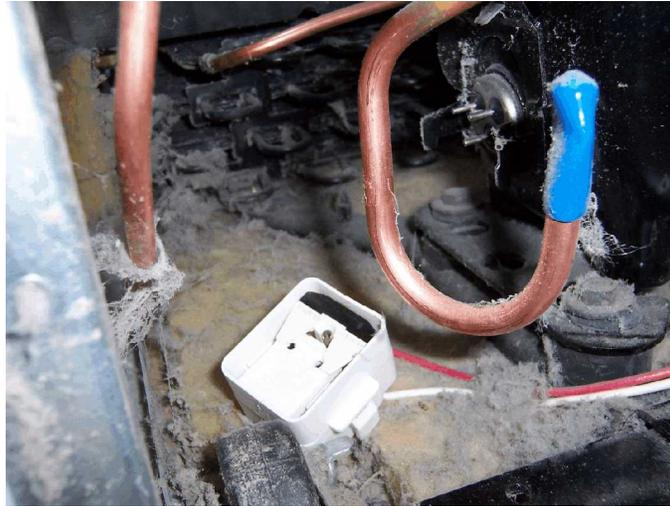
Now you have a couple of options here. You can replace the start relay with a factory one. The factory start relay will look just like the one you are replacing so all you have to do is unplug the old start relay and plug in the new one.
